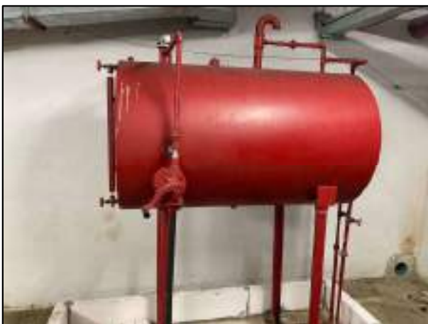
Diesel Fuel Tank of Fire pump
